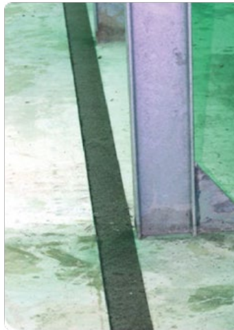
Figure 8 – Laying the bituminous strips
