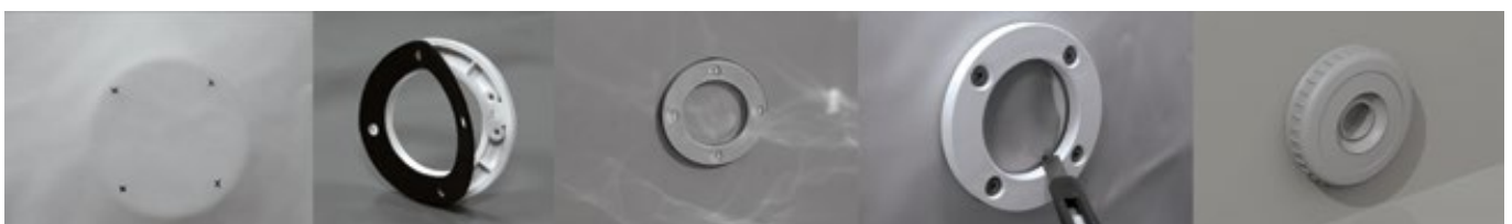
Figure 34 – Installing the return fitting flange
