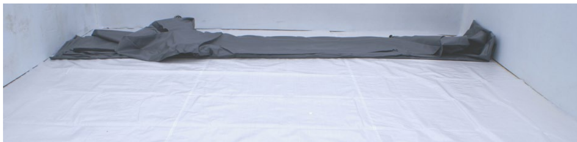
Figure 32 – Unfolding the liner
